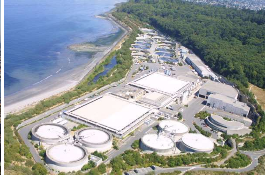
One of Seattle's Wastewater Treatment Plants
