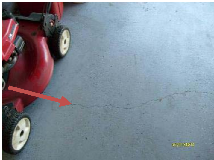
Crack in Garage Floor
