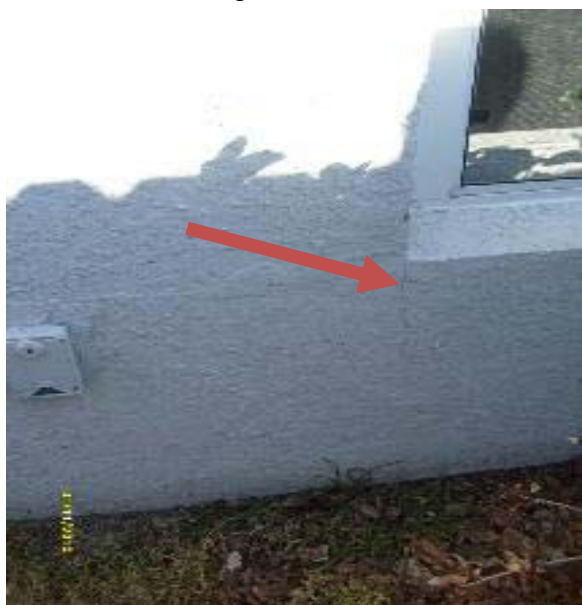
Crack in Exterior Wall
