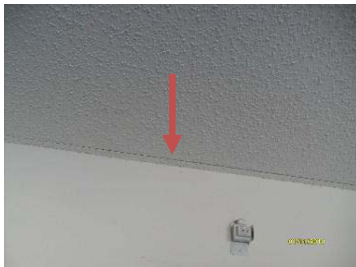
Crack in Ceiling
