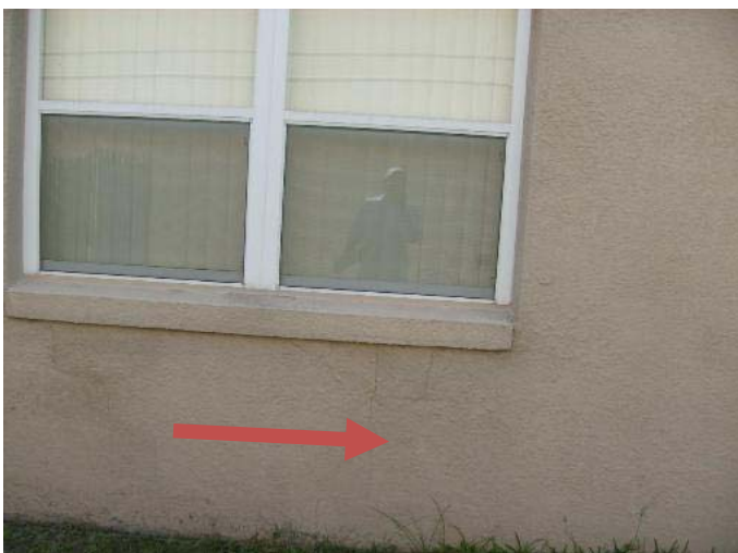
Crack in Exterior Wall
