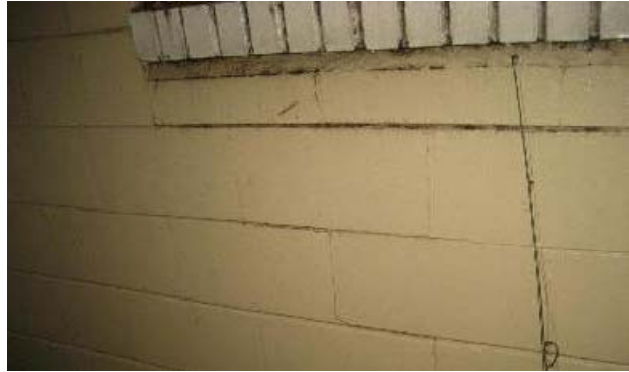
Cracks on rear elevation of dwelling
