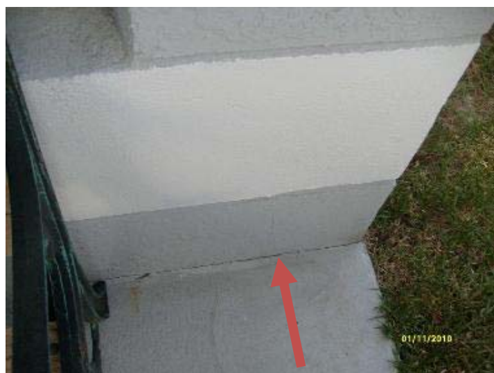
Crack in Patio Floor
