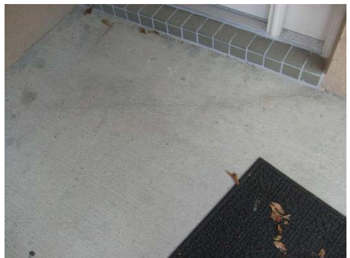
Crack in Patio Floor
