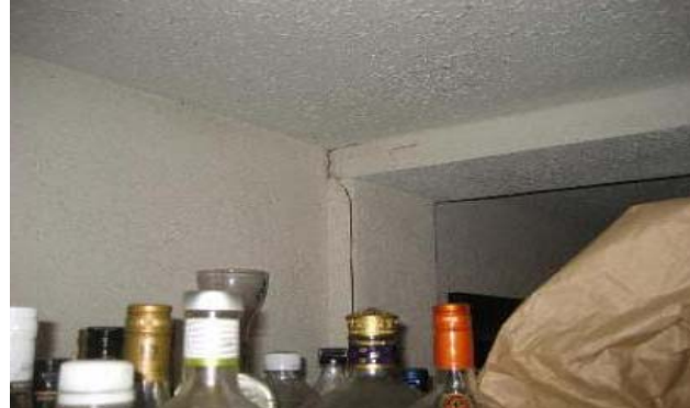
Crack at addition wall
