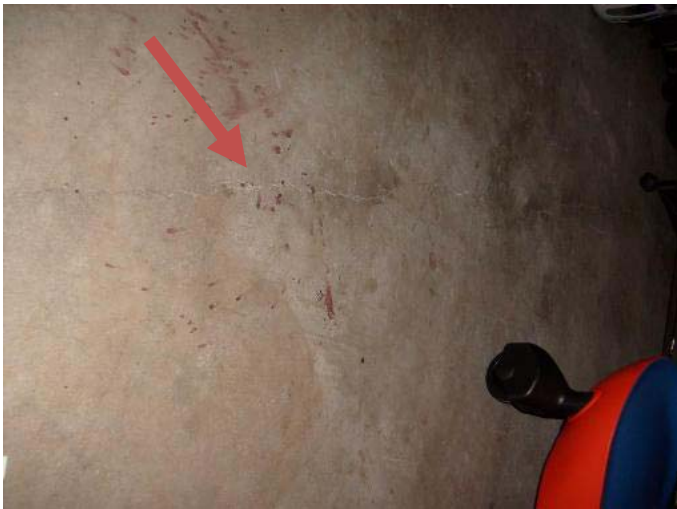
Crack in Garage Floor
