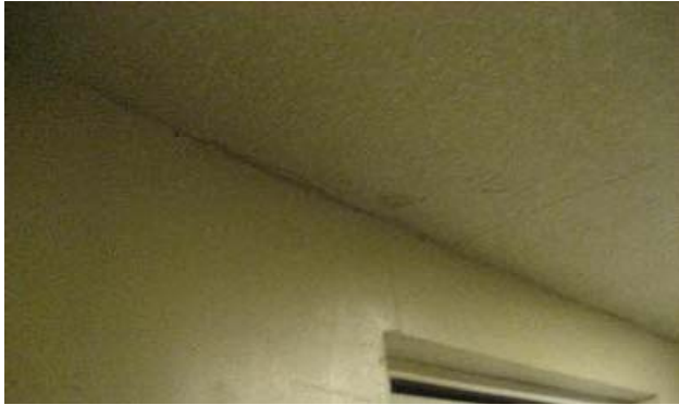
Cracks in drywall at hallway ceiling
