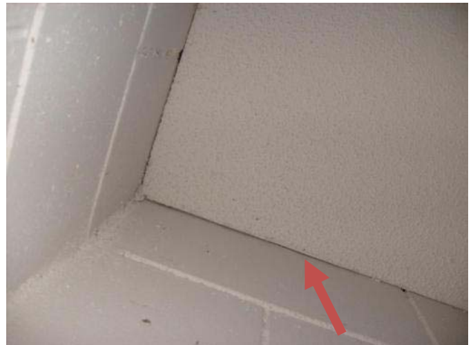
Crack in Ceiling
