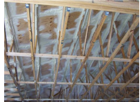
Adhesive on the under side of roof sheathing
