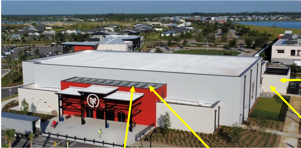
Steel Beams and Screening protect Roof Top Air Conditioning Units, water heaters, etc. from potential projectiles
