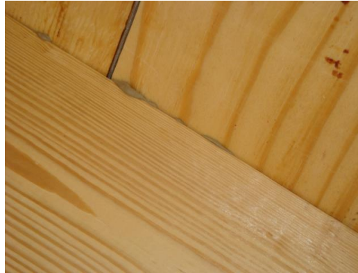
Adhesive on the under side of roof sheathing
