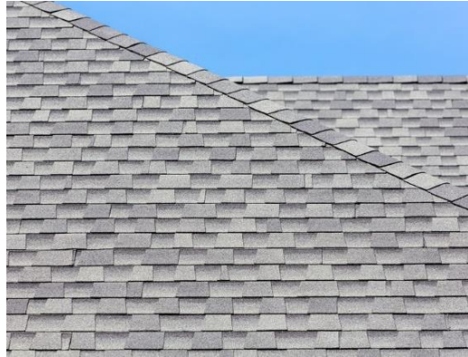
Uplift Wind Resistance - Shingles Class H Shingle 150 mph rated Class G Shingle 120 mph rated
