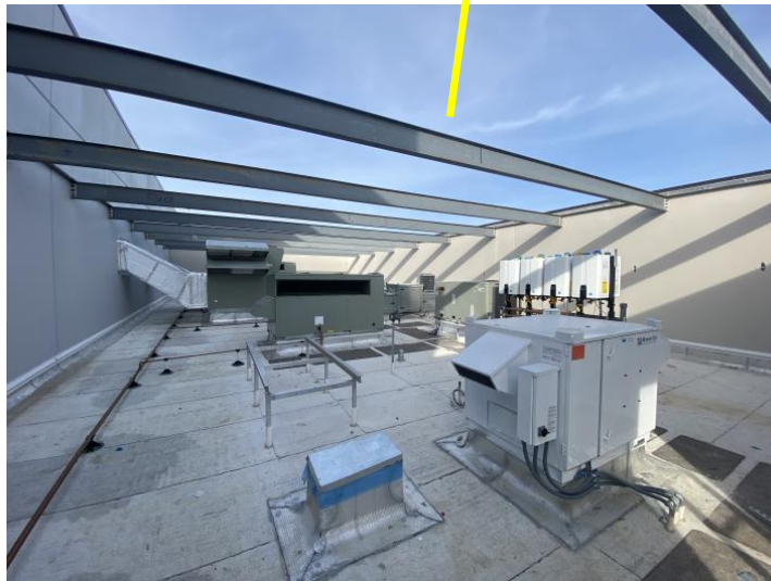
Steel Beams and Screening protect Roof Top Air Conditioning Units, water heaters, etc. from potential projectiles
