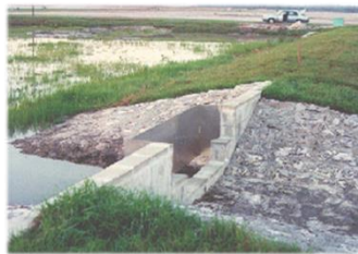
“Wet” Detention Ponds
