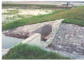
"Wet" Detention Ponds
