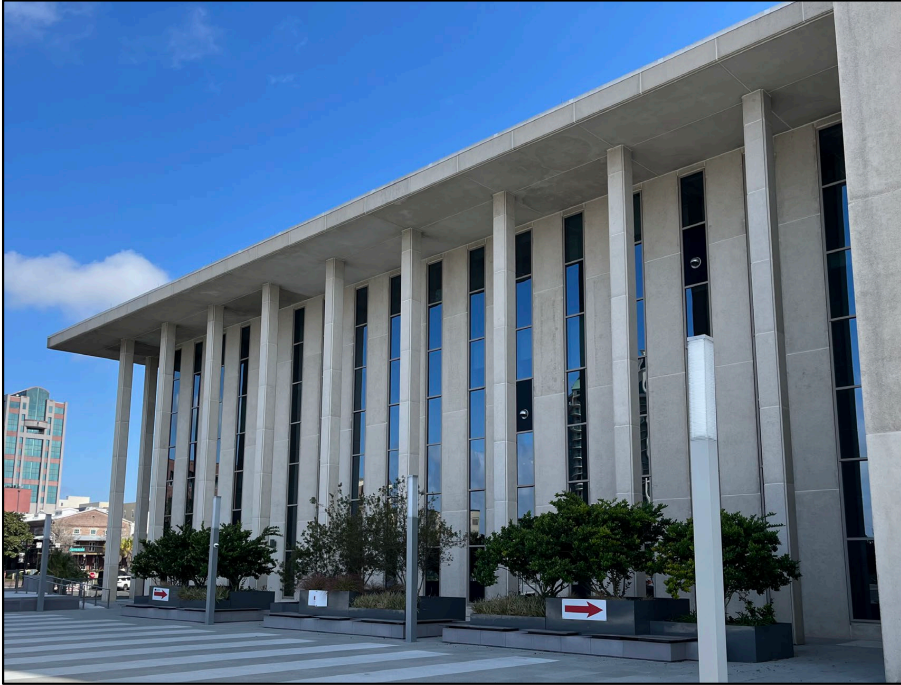
Waller Park - Capitol Building North New Windows
