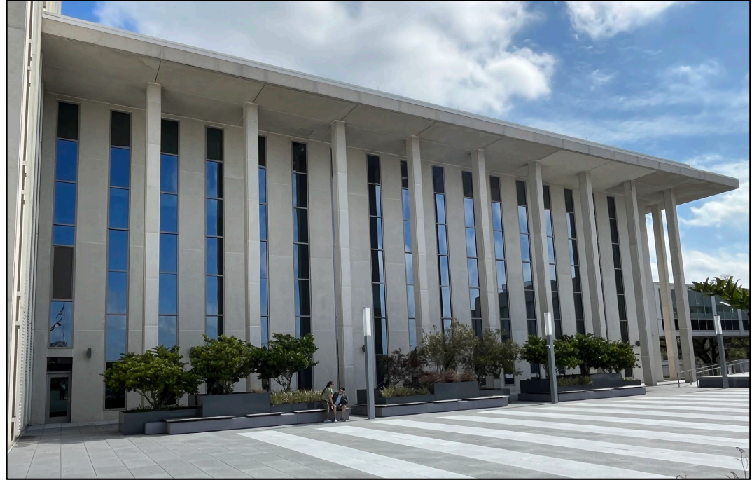
Waller Park - Capitol Building South New Windows
