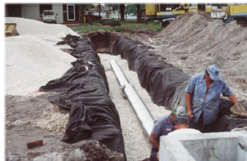
Underground Exfiltration Trenches
